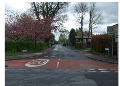
Plate 50 Excessive signage and road markings
